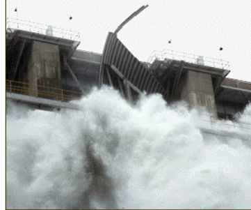
Gate failure at Folsom Dam, CA
